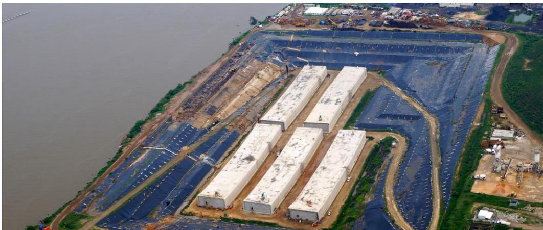
*Figure: Tunnel elements under construction*
