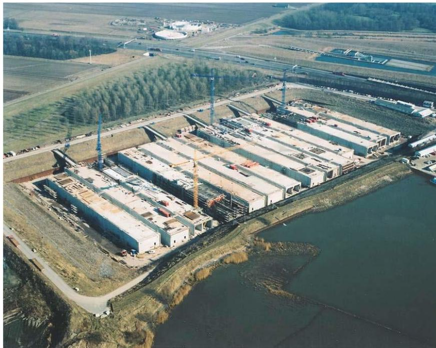
*Figure: tunnel elements for crossing with river Oude Maas and Dordtsche Kil in construction dock*
