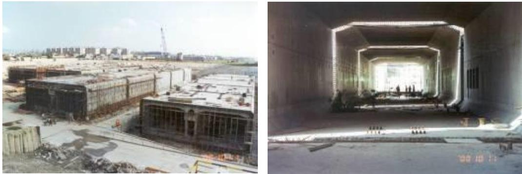
*Figure: Tunnel elements under construction*
