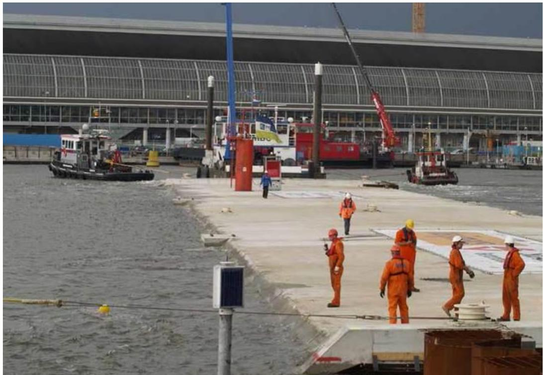
Figure transportation and immersion of tunnelement.
