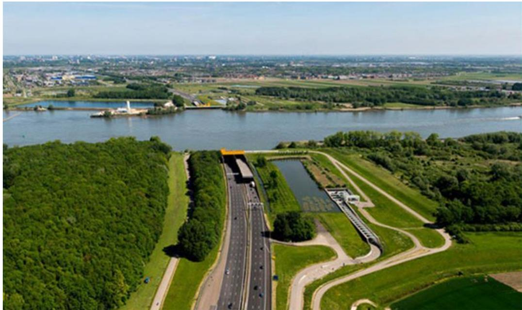
The old Heinenoord tunnel is currently being prepared for a substantial renovation and upgrading in order to meet current legislation. Next to upgrading systems and installations, a central gallery will be realized for escape and installations. It will be the first tunnel in a substantial renovation program of tunnels in the national road network in the province of South Holland. The renovation works for the 1st Heinenoord tunnel are scheduled for 2021-2023.
