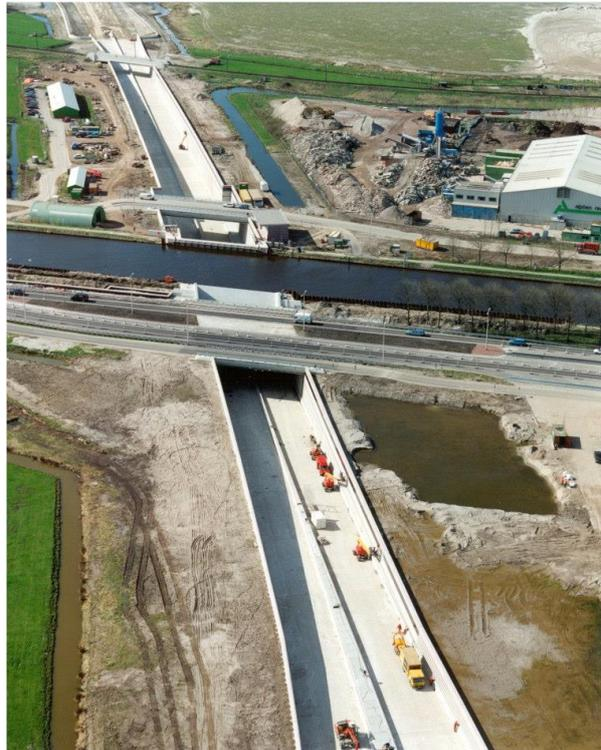
Figure: Aquaduct under construction
