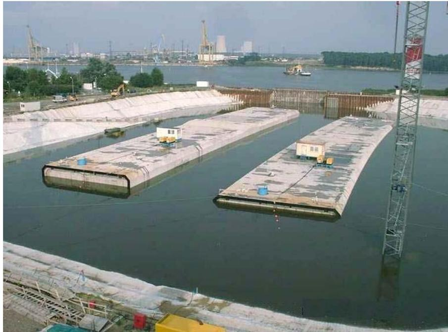
*Figure: Tunnel elements floating in construction dock*
