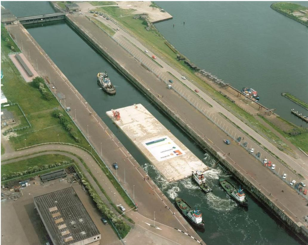
*Figure: transport tunnel elements*
