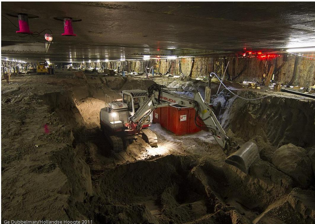
*Figure: Impression of excavation deep part of the building pit under compressed air conditions.*
