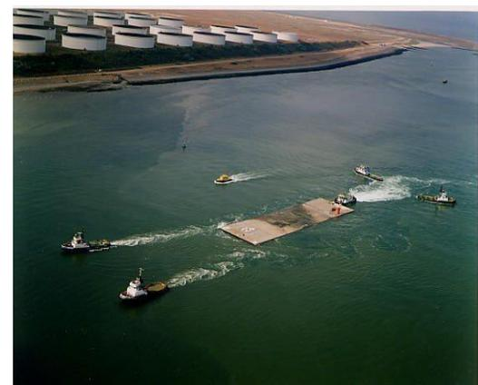
*Figure: Tunnel element during tow to site*
