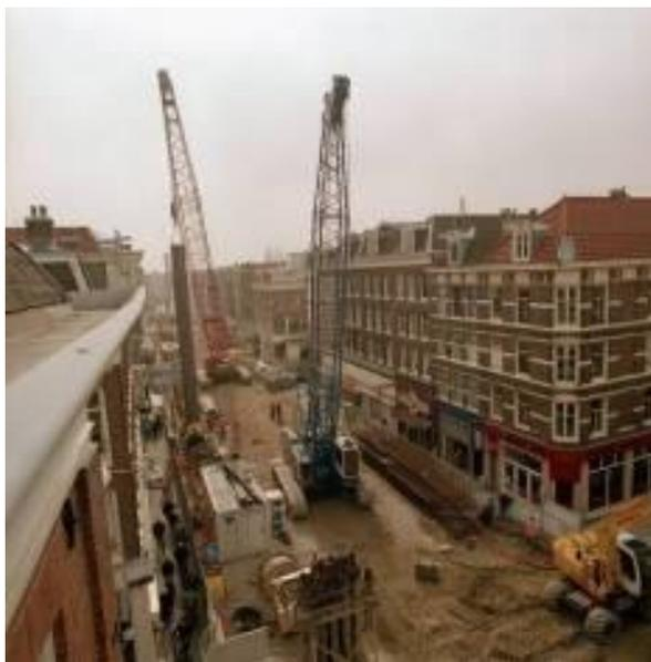
*Figure: Diaphragm wall construction*
