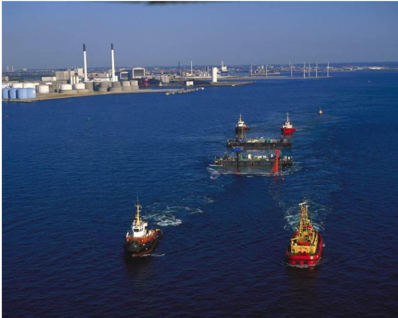
*Figure: Transport of tunnel element*
